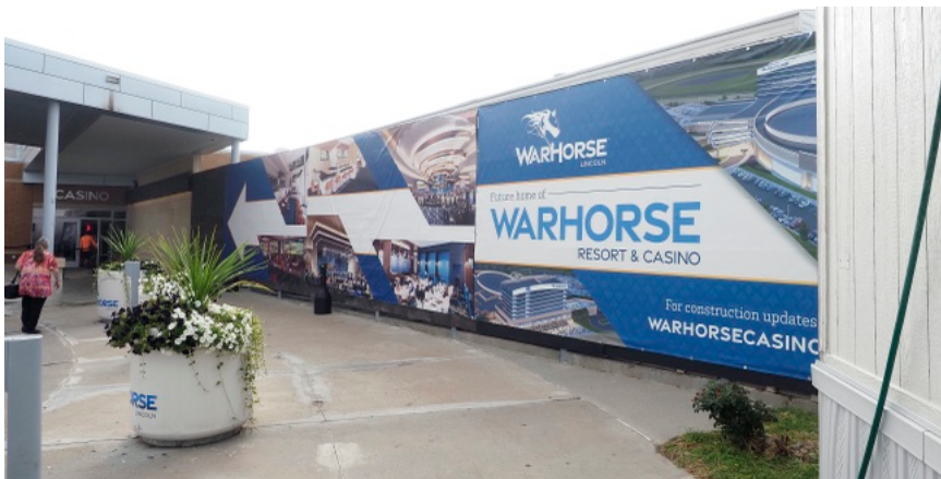
WarHorse Casino construction in Lincoln, Nebraska
